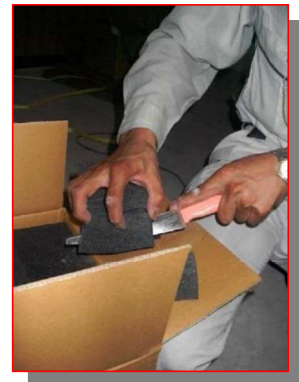
Cut into the shape of additional cables
